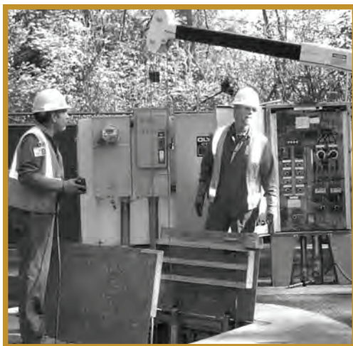
District crew repairing a pump station
