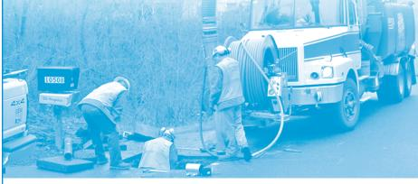
In addition to line cleaning, this truck can perform hydro-excavating with jets of water. For shallow work, the truck can vacuum soil from around a pipe to expose it for repairs.
