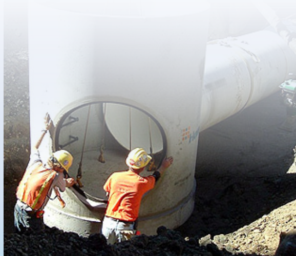
Installation of manhole for gravity interceptor
