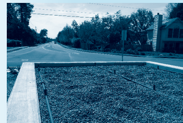
One of the biofilter beds built as part of the DCWTS project
