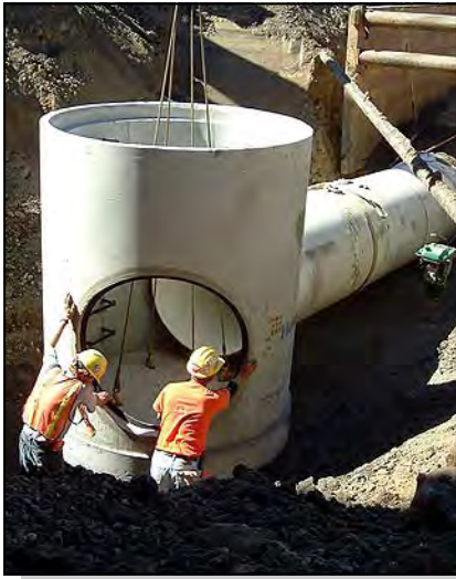
Installation of manhole for gravity interceptor – Phase 4, Segment 2
