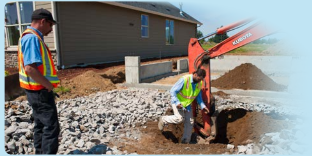
District staff person completing a site inspection
