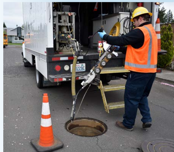
Maintenance staff inspect a sewer main
