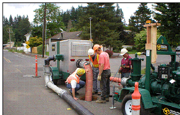
Upper Interceptor, Bypass Pump Test
