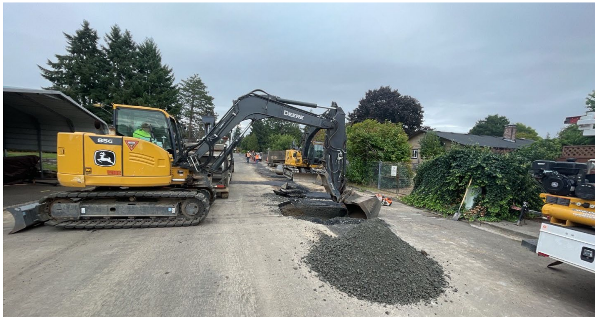
Nutter Corp. installing sewer in Sunset Strip in 2023
